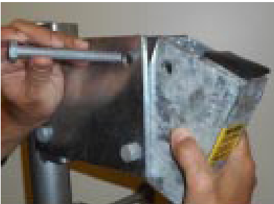
D) Insert 1/2" bolts through both sides of assembly
